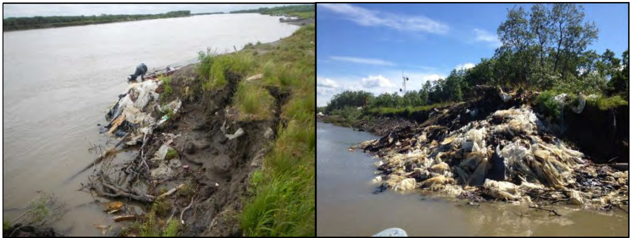
Figure 20. South Side Old Dump Site Erosion in 2012 and 2014
