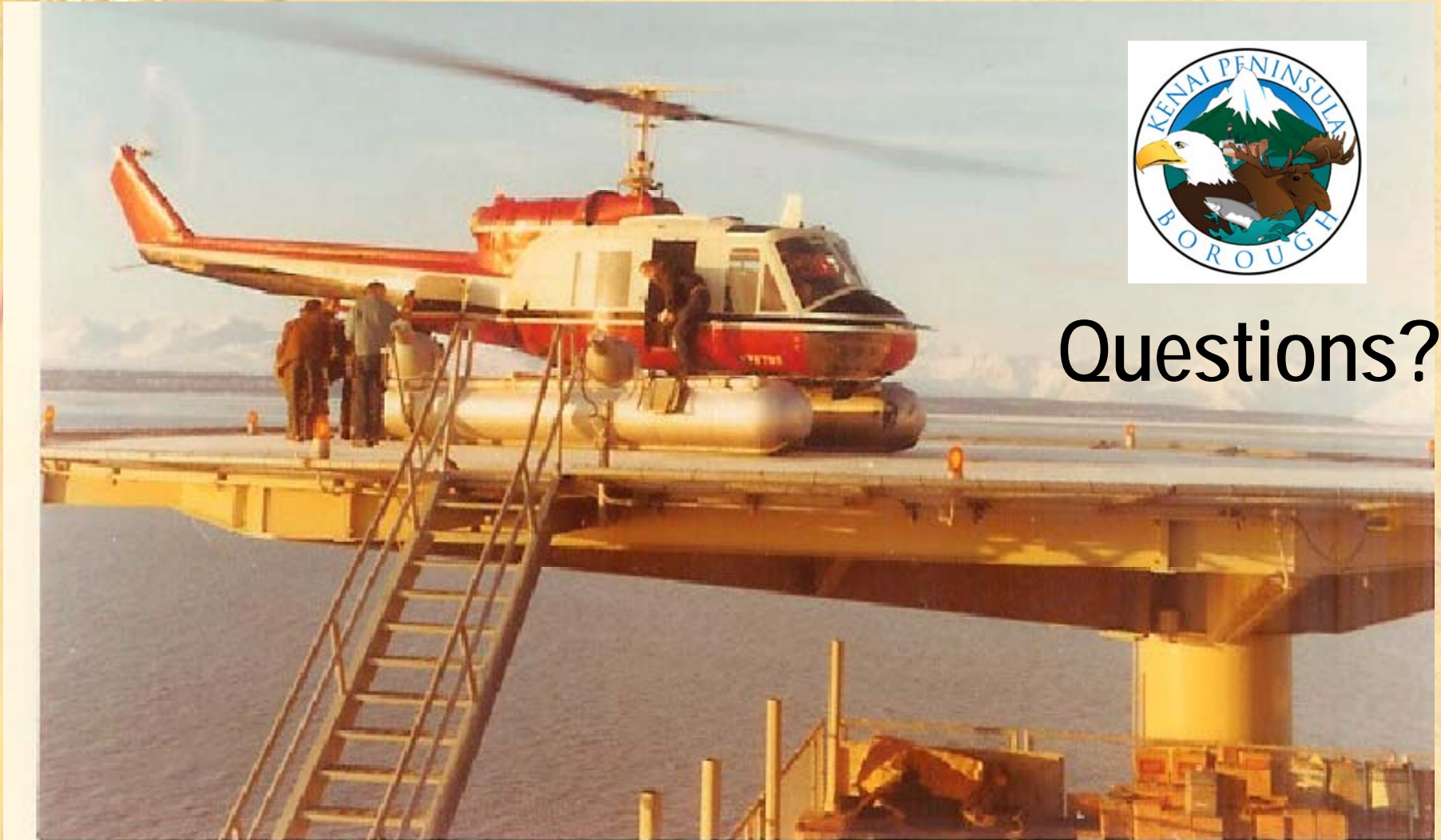
King Salmon Platform, Helipad, shortly after installation in Cook Inlet
