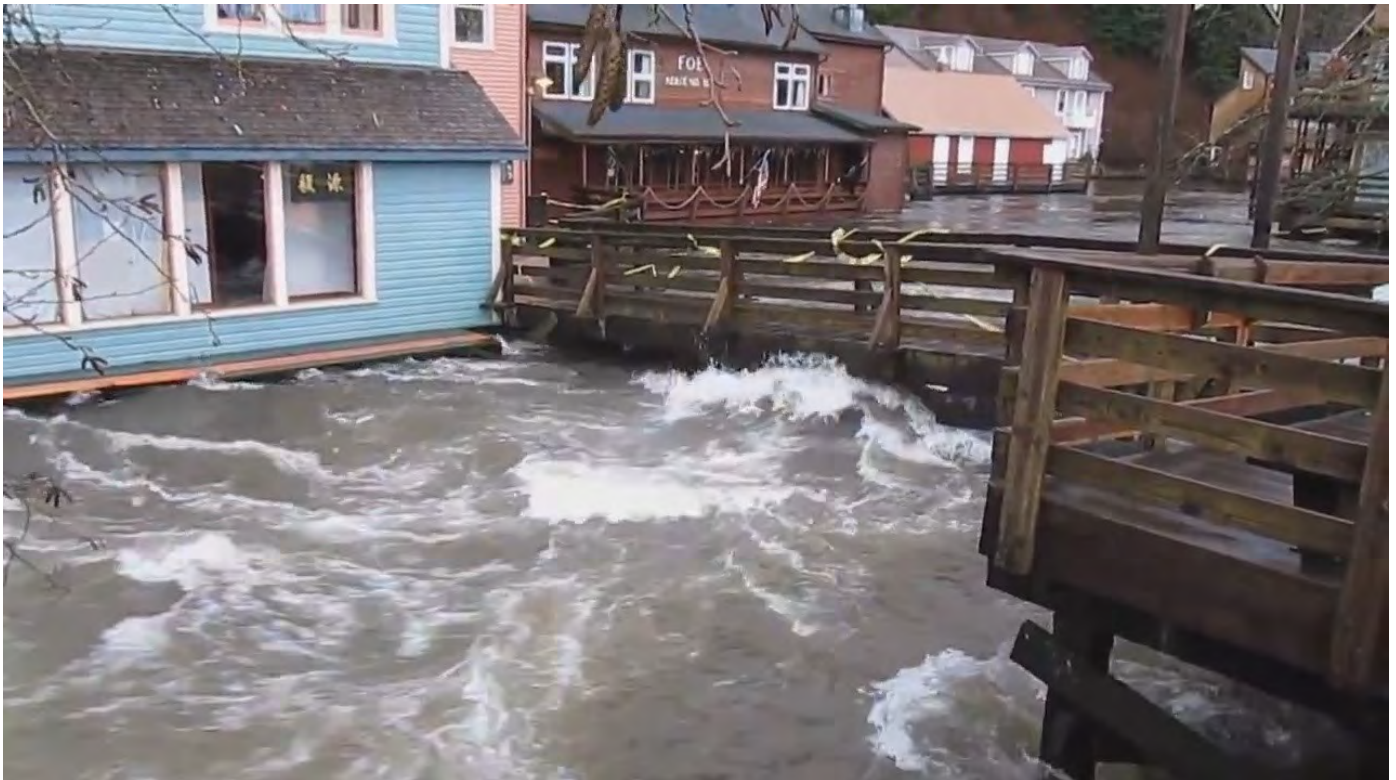
Figure 19: January 2015 Flooding on Ketchikan Creek, Creek Street, Ketchikan, Alaska
