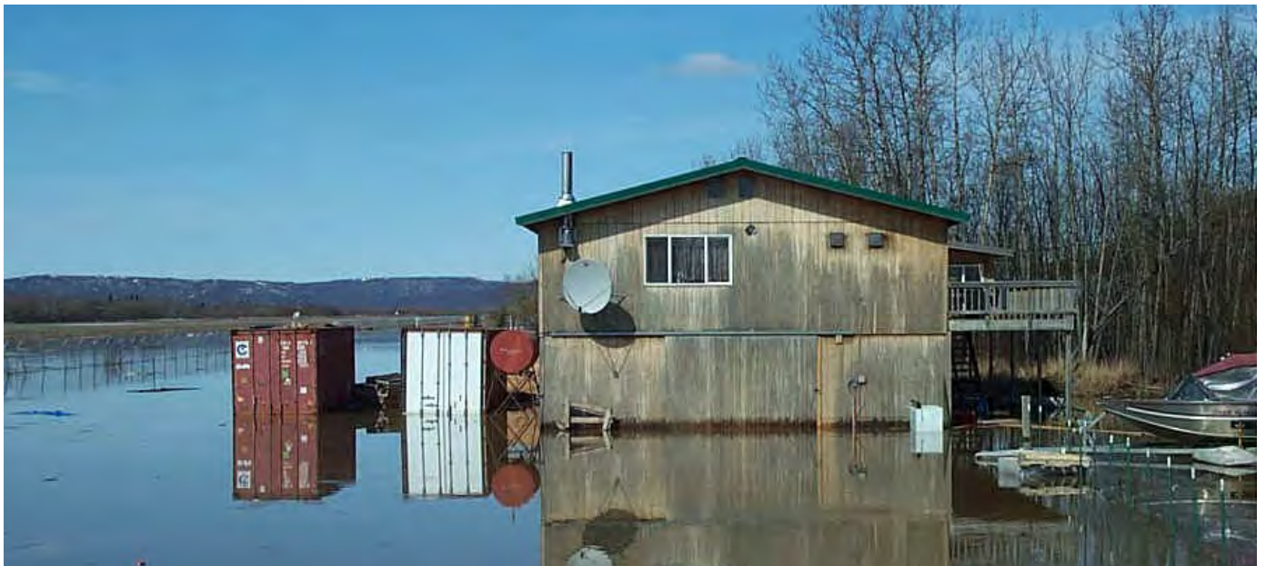
Figure 22: Flooding in the Village of Aniak
