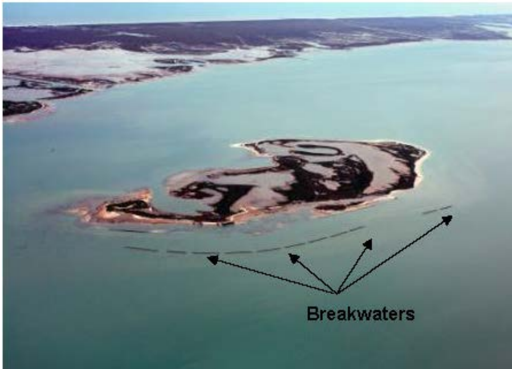
Figure 33. Example of Segmented Breakwaters
