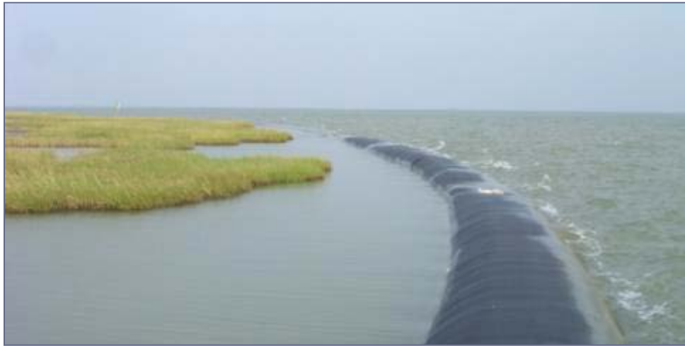
Figure 37. Example of Geotextile Tube
