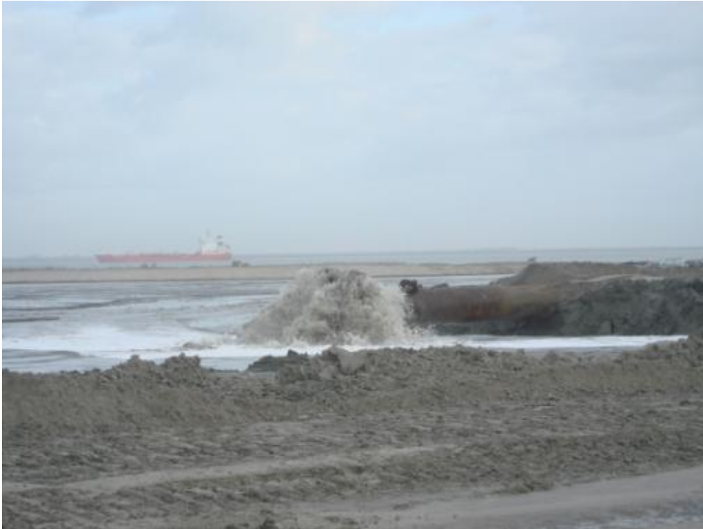
Figure 35. Example of Beach Nourishment- Discharge of Dredge Pipe
