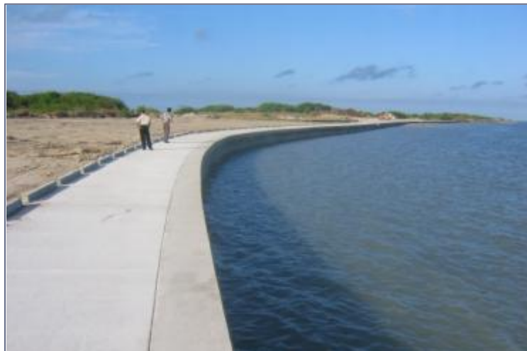
Figure 36. Example of Concrete Panel Bulkhead with Sidewalk
