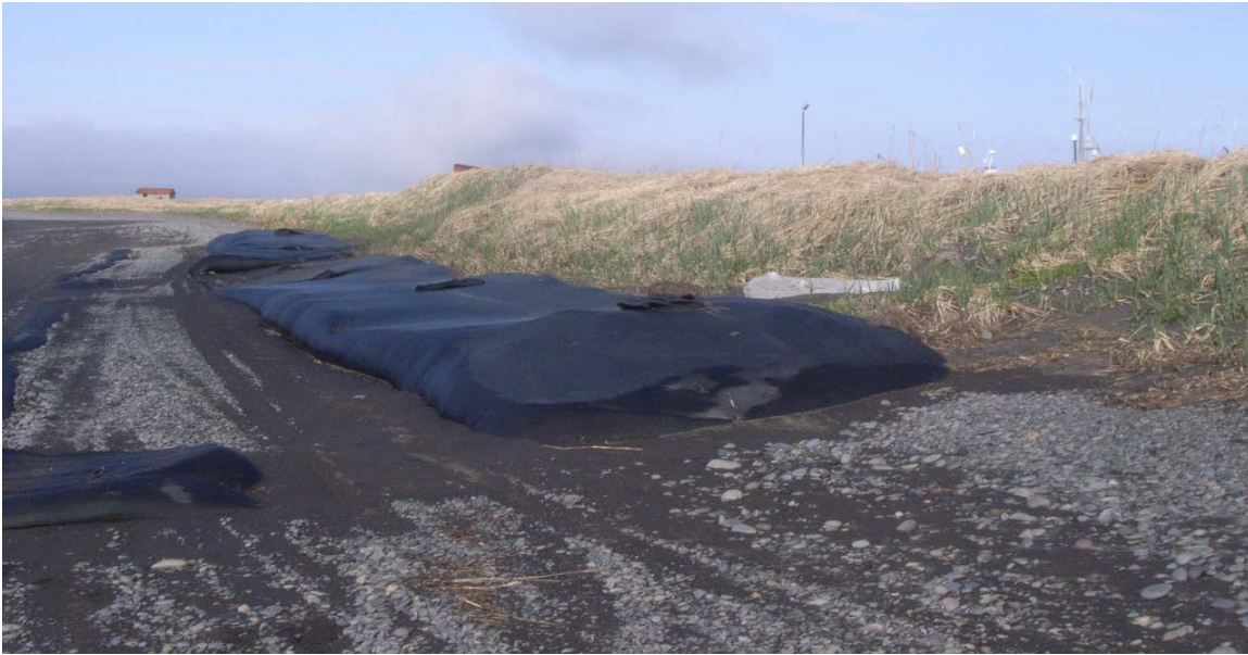
Figure 24. Geotube Containment Structure
