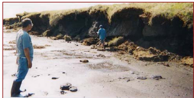
Photo 4. Undercutting effect of Ninglick River at low tide.
