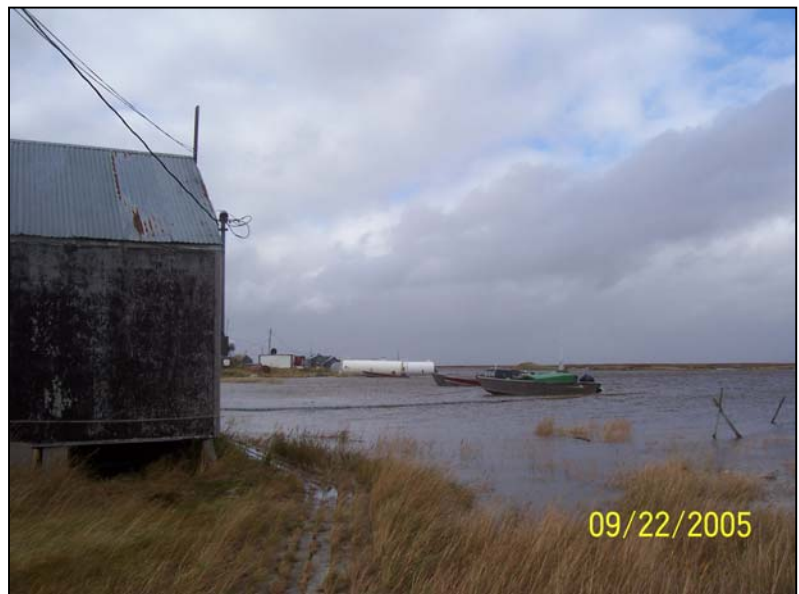
Photo 6. Shoreline erosion in Newtok.
