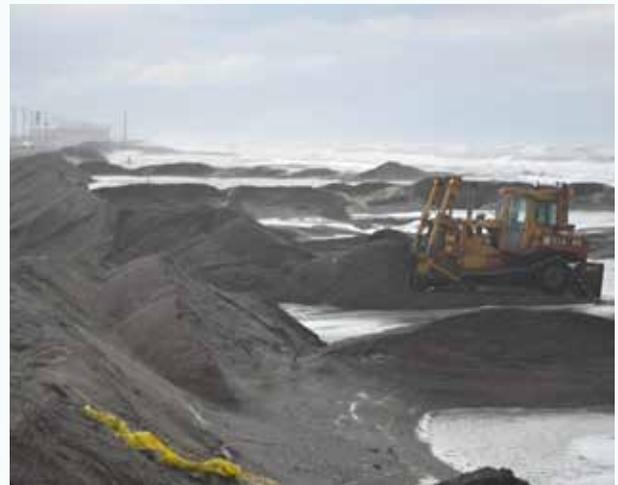
**Figure 44:** A five mile gravel berm provides insufficient shoreline protection from coastal erosion in Utqiagvik and must be repaired after every storm, as shown above, which costs \$8.3 million annually. The U.S. Army Corps of Engineers project will construct a fortified rock revetment to protect the shoreline. **Credit:** North Slope Borough.
