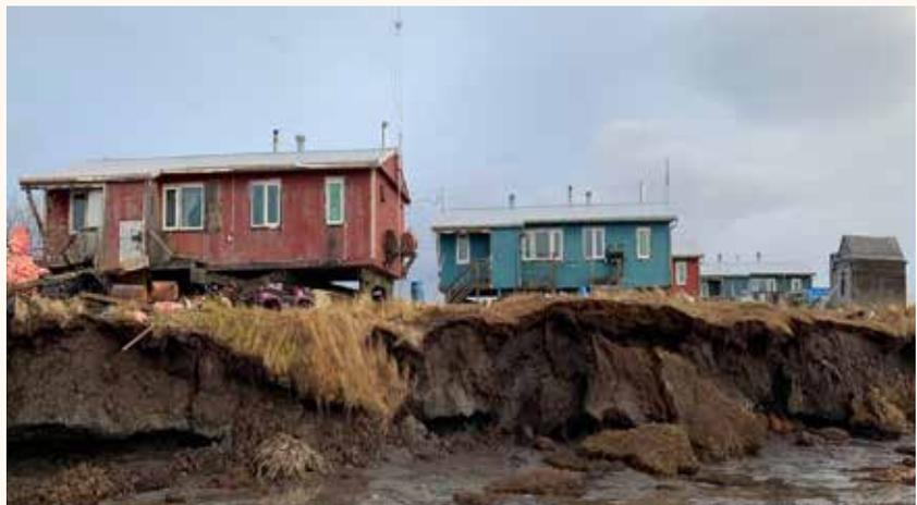
**Figure 18:** *The eroding riverbank (shown above in 2018) forced Newtok to demolish these homes in 2019 to prevent them from collapsing into the river. Credit: Andrew John; Village of Newtok; 2018.*
