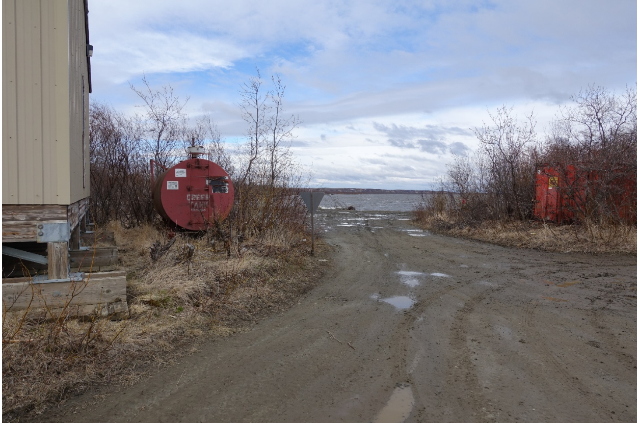
Figure 8. Armory building and road leading to boat and hovercraft landing area. May 11, 2018
