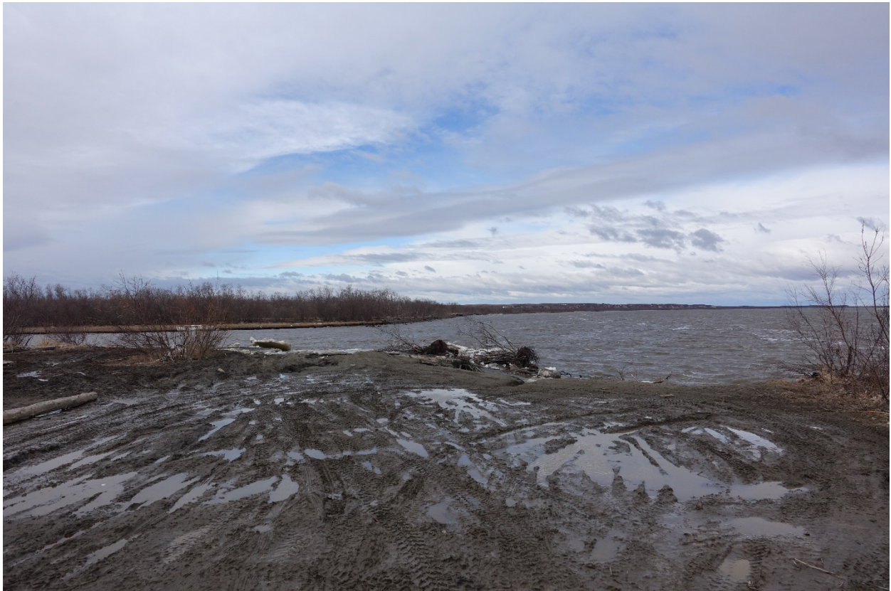
Figure 9. Looking southeast at the damaged boat and hovercraft landing. May 11, 2018
