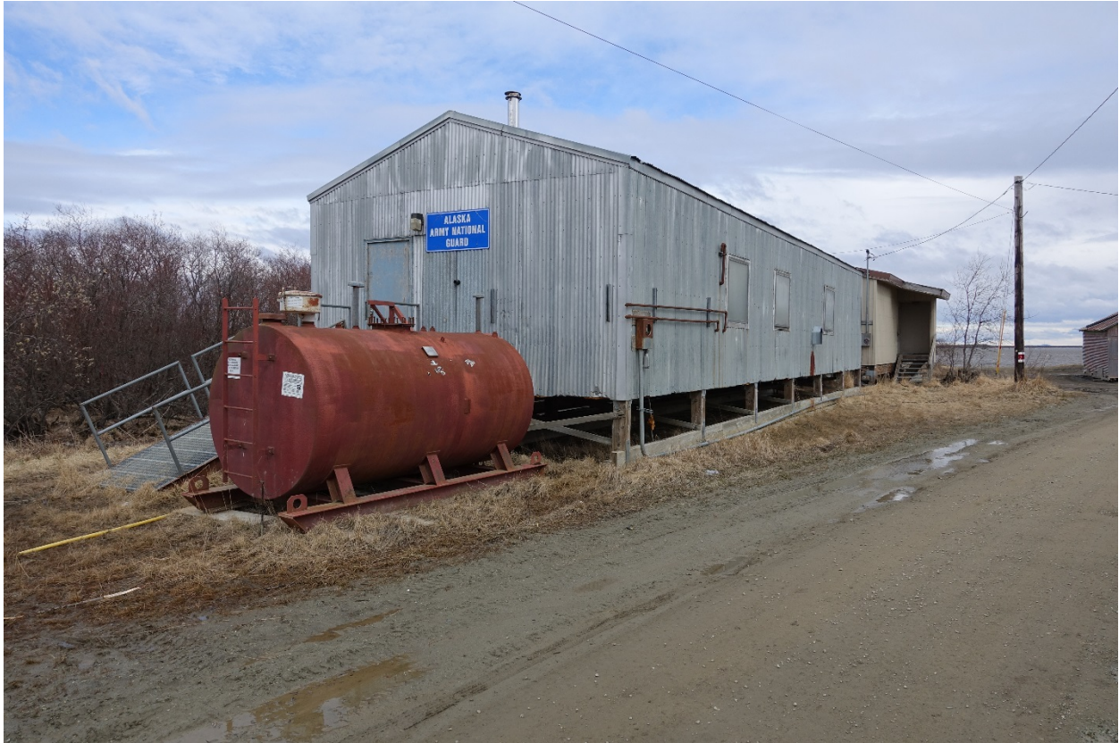
Figure 7. Armory buildings on May 11, 2018. Note the Kuskokwim river in the background.
