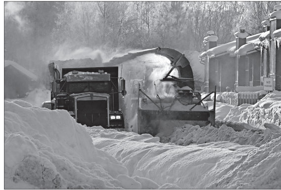
A snow removal and street-widening operation on Pioneer Drive in Muldoon on Wednesday.
